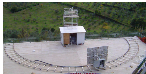
Solar power testbed in Italy.
